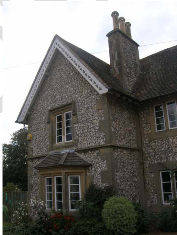
Chailey Church of England Primary School with its field flint facade
