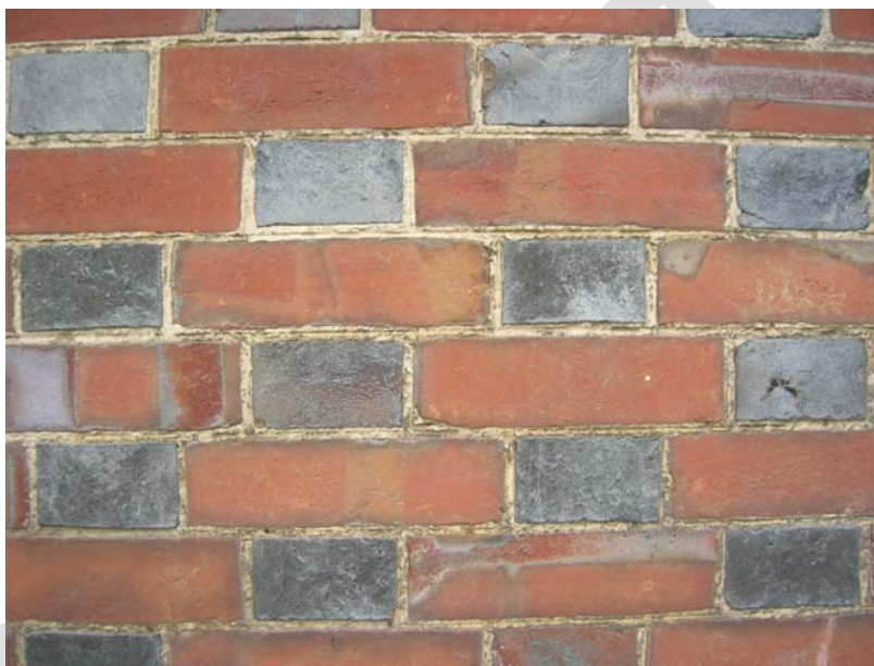
Example of the use of vitrified headers within Church Farm Cottage
