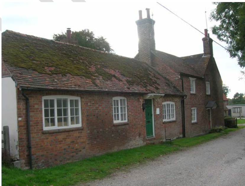
Relationship of Church House Cottage and Church Farm Cottage with Church Lane
